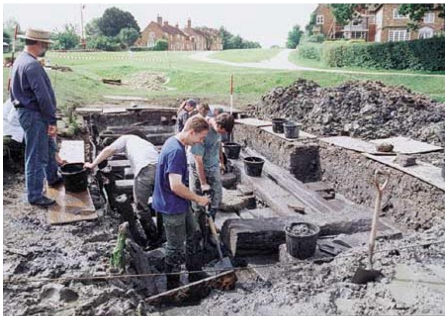
Plate P7e Excavation at Bucklers Hard showing the well preserved timber below the silt
