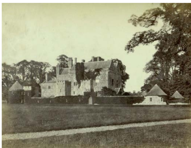
Photograph around 1865 of west and south facades showing turrets
