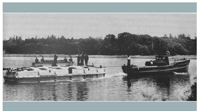
A basin was dredged at Clobb Copse for constructing concrete floats (shown left in the photo) to support roadways across water. 470 of the floats, known as Beetles, 50 from Beaulieu River, were towed to the coast of France. They supported roadways over the sea to Mulberry Harbours used for the Allied invasion of Normandy in June 1944.
